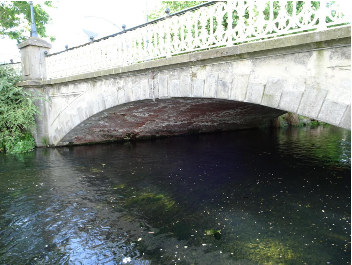
Bridge D is another brick arch and this one is skew.
