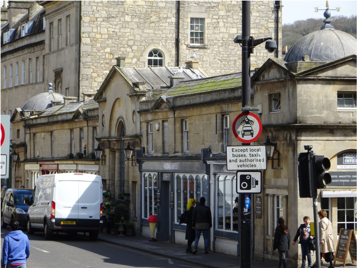
Forsyth also tells us that “in 1792 Thomas Baldwin added a storey. For a while, I thought that was just squeezing a floor into existing space but looking more closely, the pavilions and central section could all have stopped at the first frieze and the rest of the building at the top of the shop windows.
