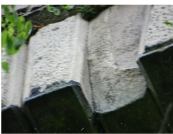
I have deliberately shrunk this to disguise the poor focus but it is good enough to see that it is almost certainly a fault in the stone. It just happens to occur in four voussoirs closely spaced.
