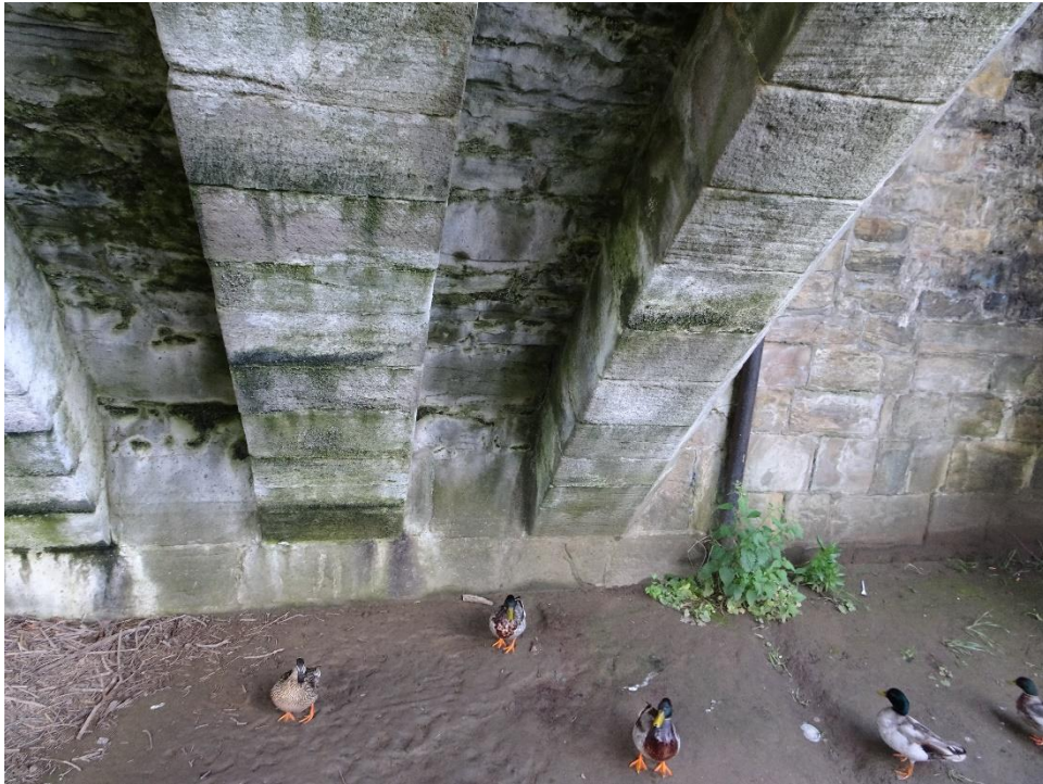
Beyond the join the stones are much larger, but the joint is actually visible here and the rib at the olde edge (right) is square edged.
