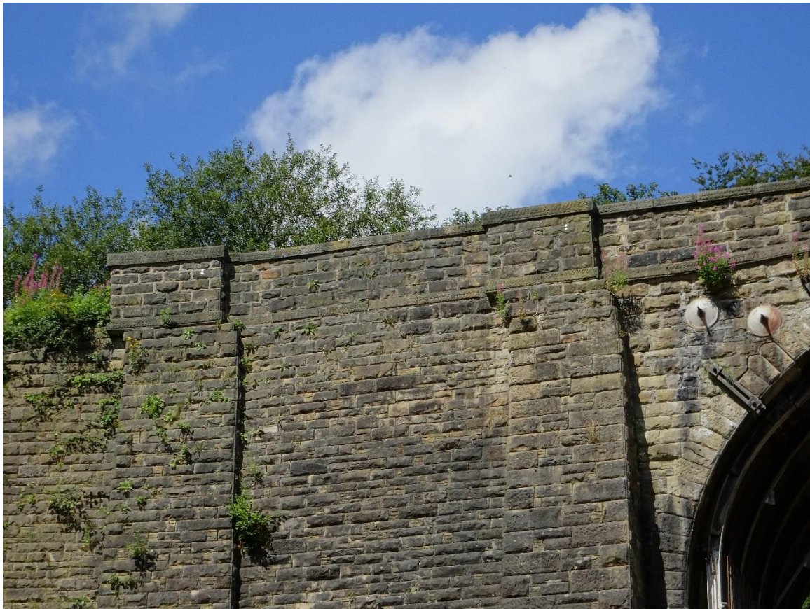
And the massive joggles in the top of the pilasters.
