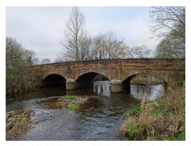
Looking through the right hand span we see an island with a modest flow against the near bank and a much greater at the far side. Downstream, there is another, very shallow, island which blocks less of the main span. Looking more closely, we see that in this, relatively gentle flow, there is a substantial flow across the upstream edge of the pier where any scour is likely to be most severe.
