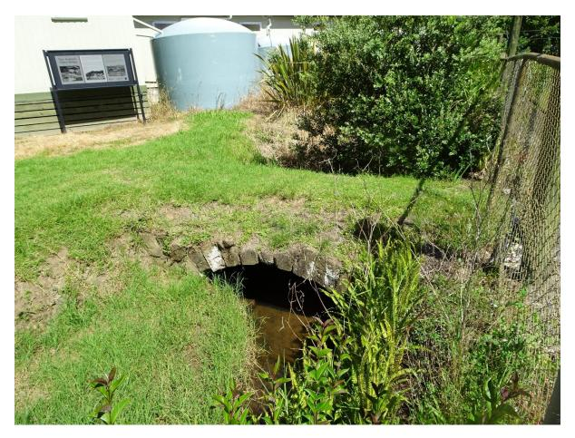
The arch evident here is very much less of a curve than the original which I suspect was semi-circular or very nearly so. The lake shown in the 1860s photo obviously silted up long ago. Note that the elevated viewpoint marks this as the upstream side.
