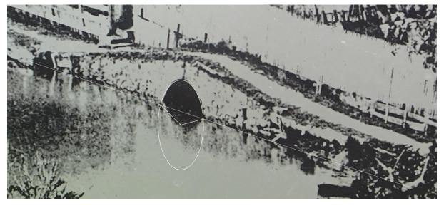
Stretching the ellipse shown here till it is a full circle gives the angle above water level as 144degrees.
