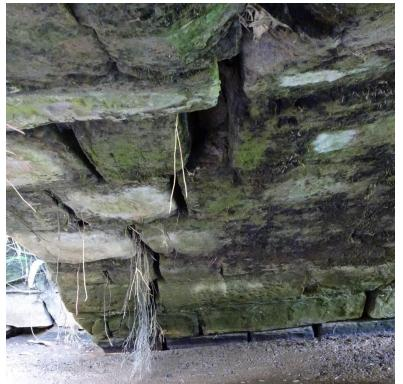
The crack at the upstream edge follows a similar pattern. Much wider at the crown and moving towards the edge at silt level.
