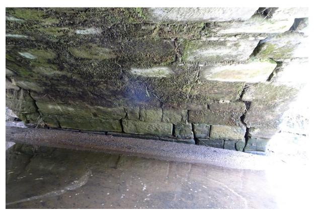
Here we see the northern half of the arch and it is immediately obvious that the curve continues into the silt. There is a substantial crack/joint opening at both edges, the right hand (downstream) one is most visible. It is much wider at the crown than at the end and moves steadily out towards the edge at the end as well. This is surely caused by pushing out from the crown.
