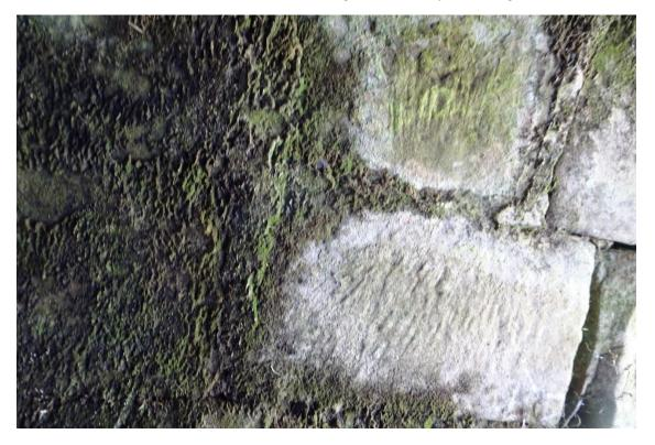
Even through the vegetation we can see that the mortar spreads across the face of the stone. This is probably "as built". The mortar will naturally spread across the centring as the bridge is built. The fact that it still does so reinforces the view that floods are rare.
