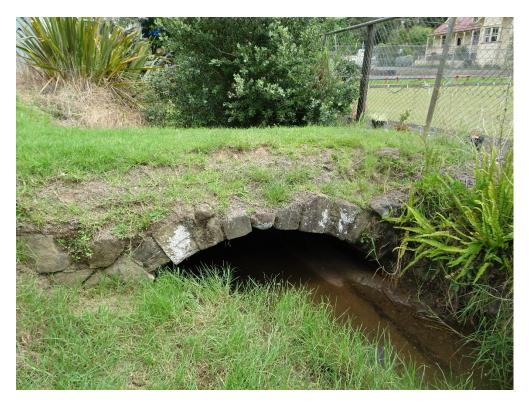
The spandrel walls and low parapets are long gone but it is interesting that the walls remain below arch crown level which is probably the top of solid backing. Did the quarriers take a clue from that or were the stones just better fixed?
