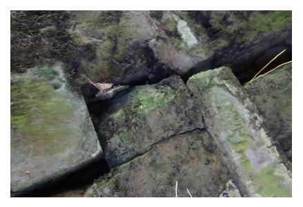
The upstream edge of the bridge is at the top of this picture and these stones are close to the arch crown. Note how that split stone bridges between the two sides and is set to become a jack, pushing the sides apart with even modest shear movement.
