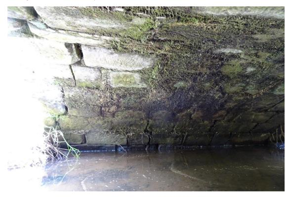
The south end of the crack is similar in form, though it seems to pass through at least one stone.
