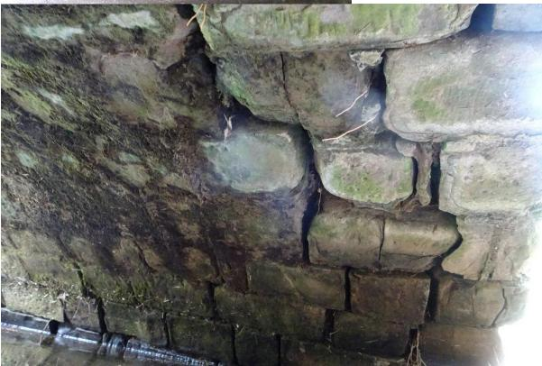
The south end of that crack is quite spectacular. It divides into 3 making it difficult to judge the width but it also passes through some stones. Here there is still mortar in some of the open joints but much of it has been washed out, presumably with water from above.
