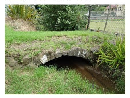
Finally, a look back on top. Note how thin the grass is on those sloping sides and how thick on top. The sides are clearly eroding faster than the grass can grow. There is very little cover left at all above the major cracks, but I suspect the soil slipping is part (along with mortar washout) of the cause for the width of these cracks.
