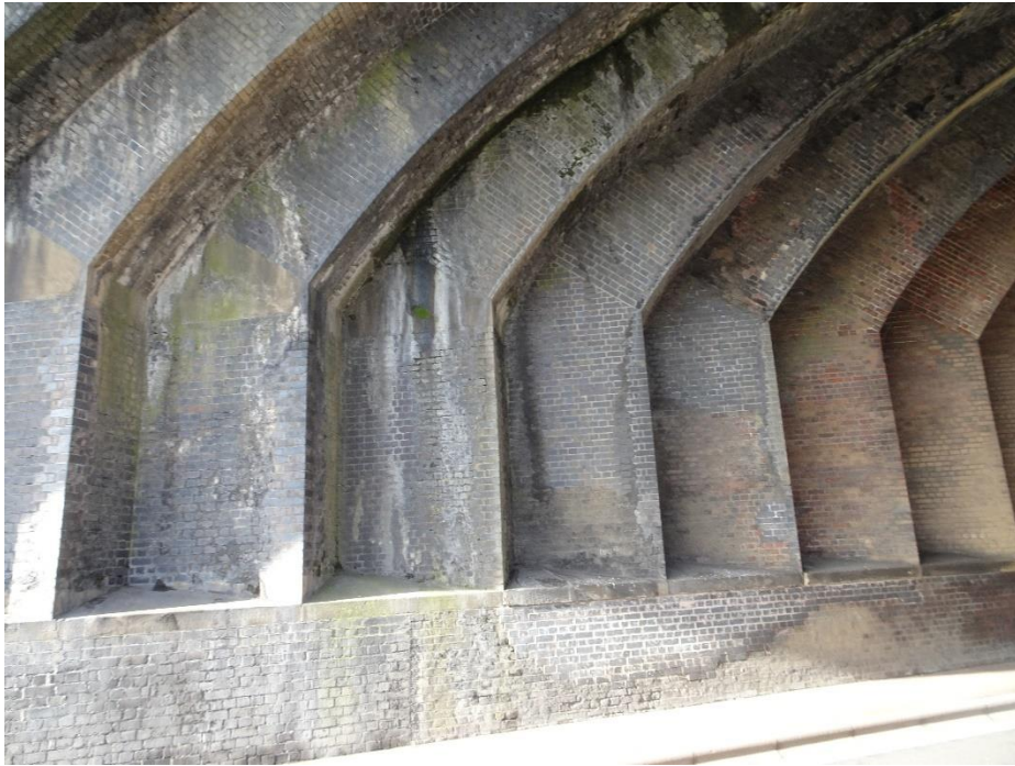
In this closer shot, the water running down the skewback has obviously tracked down from higher. The run naturally hugs the intersection.
