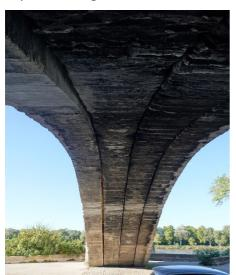
The end span (left) looks rather less happy, having suffered repeated attack by motor vehicles. I suppose it gave as good as it got, but has this been enough to drag the leftmost ring away from the rest? The wide joint (enlarged below) is stuffed with corrugated pipe and expanding foam. An unsympathetic treatment perhaps intended to stop fill material (right) dropping through.
