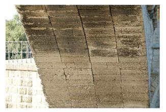
There is a definite tendency for the separate rings to separate at the crown. That this separation is so
