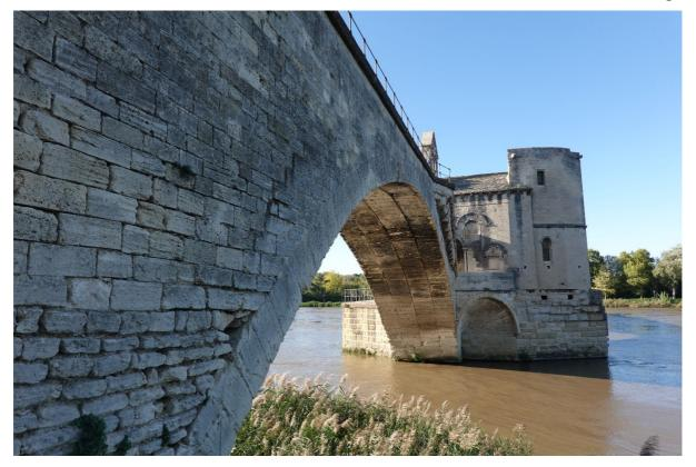
Close inspection reveals that a single course of three longer stones provided some bond at low level. At the river bank (right, viewed from the chapel pier) these have fractured at the main joints. At the chapel end of the same span (below) the damage is less complete and the distinct course more obvious.
