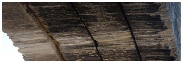
Where that fill is visible from the footpath, as above, it seems to be in the form of quite small shards of stone with no mortar, so the fear of pieces dropping out is not unfounded.
