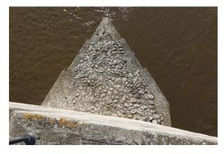
That outer ring is much less eroded than its deeply-grooved neighbour. It also sits lower through most of the span. What is going on? My first thought was that this was something to do with the plan step at the river end of this span (below). But that goes the wrong way!
