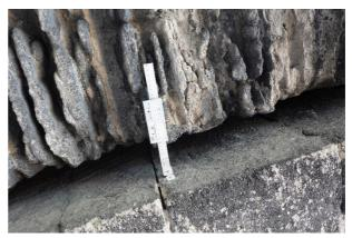
take the liberty of tensioning the tape to check the current reading, so it might not be indicating a 0.5mm movement in two years as it appears.
