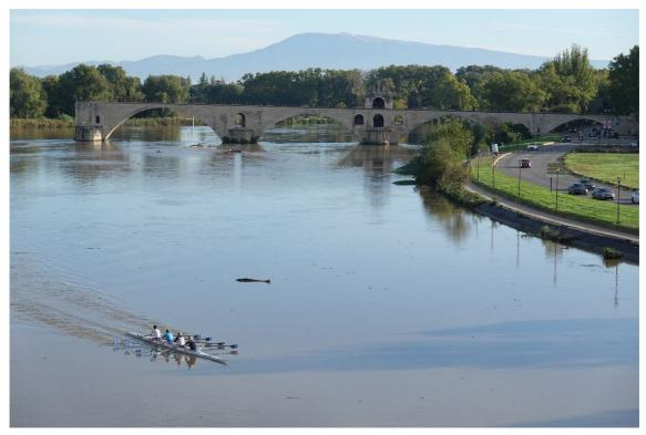
The end span stands happily, indicating that the piers, though very much narrower as a proportion of span than those of many medieval bridges, are wide enough to act as full abutments. Each span is an independent bridge.
