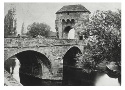
An 1866 photograph shows both passageways and the downriver widening clearly, and the parapet line on the upriver side does not seem to deviate, so the widening is surely present there as well. The bridge now is little changed from this view, apart from local repairs.
