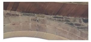
The replacement arch has an open crack at the crown. This crack should give anyone working on under-ringing an arch pause. There is no thrust in these voussoirs; they must be hanging on the mortar above. If that mortar let go, they would drop into contact, so this isn't dangerous, but it isn't what was expected
