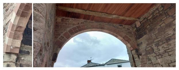
The arch over the road on the Overmonnow side of the gatehouse was rebuilt relatively recently in freshly dressed stone, but it was in place for long enough to accumulate lots of impact scars. It is dated 1989 (I think) on the inside face. The road was finally closed after construction of a new road bridge in 2004.
