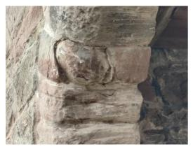
The gatehouse has suffered badly from vehicle impact over the years. Coflein <u>has images</u> of the town side arch knocked out completely, with the remaining masonry arching to the upper window. The voussoirs on this side are still have very rounded corners, perhaps the arch was rebuilt from the existing stones.
