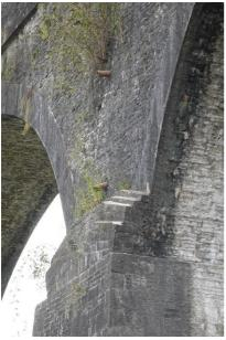
Zooming in a bit closer still (left - the Sony RX100 I inherited from Bill is a phenomenal tool), it looks distinctly as if the rubble of the ring extends out further as the outer voussoirs step out. The face of at least one lower voussoir has spalled off, perhaps as the less rubble masonry has compressed slightly relative to the stiffer ashlar. The corner of the pier seems to be having some trouble too, what is driving that?
