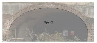
The common case in assessment is that we have a measured span and rise and we can see the springing points. In this case, if we have a photo from close to mid span and now too far below the level of the arch, it is very quick to check whether the shape is elliptical
