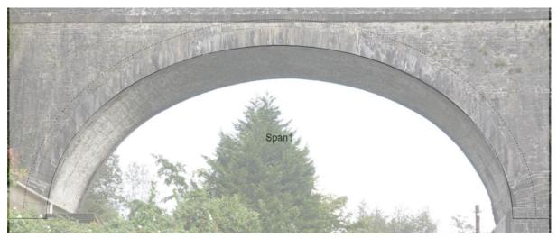
From which, we have a revised though partial view on the geometry. The span:rise ratio might well be 3:1, but we can't be sure without measurements or a square on photo.
