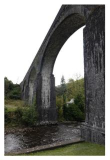
The views from below are dramatic. The view left shows how slender the superstructure is in plan. Notice the lime staining from the rubble ring continuing down the pier, where the dressed edge voussoirs are clean.
