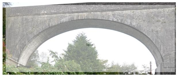
That's an interesting result. The Archie-M curve drops below the real intrados to the right, but it's much closer at the left. I guess that is a result of perspective distortion in the image. Compare the ring thickness drawn by Archie-M with actual ring in the photo. The Archie-M ring thickness is too large everywhere, but it is better at the right than at the left. Again, the difference is perspective.
