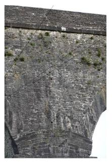
I left struck by the scale of the arches, but the shape was also unusual. Clearly not segmental, the curve is presumably either elliptical or multi-centred. In training courses I point out that the eye is remarkably sensitive to the abrupt changes of curvature of three-centred geometry. The rarer cases with five or more centres have subtler changes and will be less obvious, but we can generally see the difference between a three-centred curve and the continuous change of an elliptical curve.
