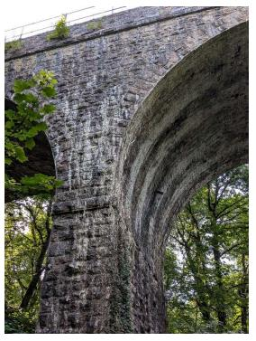
Waterproofing is never perfect, and over 150 years, water is likely to find routes through it. We often see water or lime staining starting at well defined levels, which gives evidence that water is ponding there and finding a way through the masonry. There is some evidence of that in the pier faces. The line isn't perfectly well defined, but it doesn't disagree greatly with the drain.
