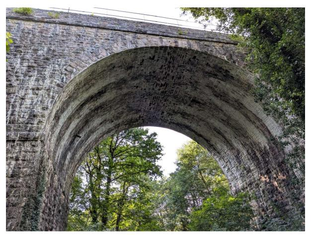
The most striking thing about this structure is how thickly encrusted with carbonate deposits it is. These have layered over and through ivy growth to remarkable effect (right).
