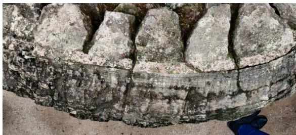
which gives a great view of internal construction: rubble concrete with a pretty ashlar skin. This was very well built, with much more mortar than I would expect to find in most mass masonry.
