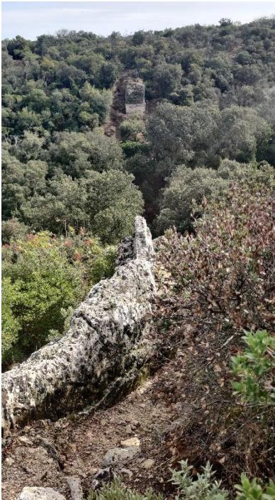
The construction of that curve (on the cliff top to the south of Pont du Gard) is fun, making the most of natural rock and using wedge shaped stones to form the curve.
