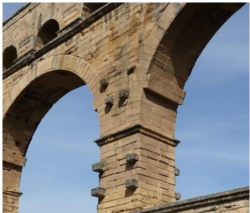
The original piers were built with normal bonded masonry. In the second pier above, the ledge appears to be lower and below the arch springing, but the stones are bonded up to the same level as in the near span.
