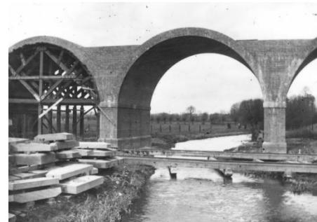
The thrust from a single strip of a third or a quarter the full width, in contrast, exerts thrust in proportion to the width. By advancing strips of arch in a wedge formation, the piers are protected without tying up two full spans worth of centring.
