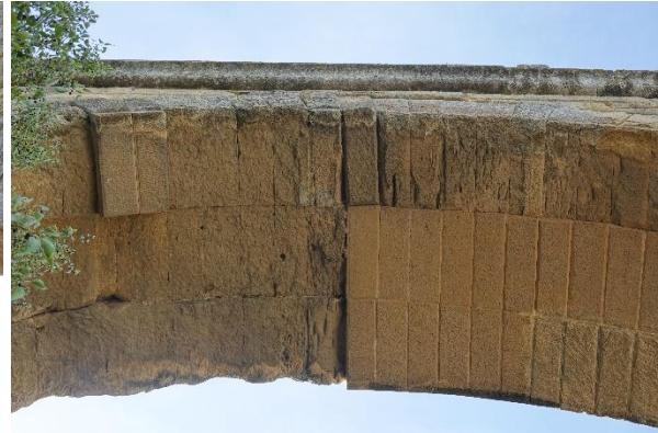
Repairs to the upper, aqueduct tier have been more extensive. I suppose the small-block wall is repair.
